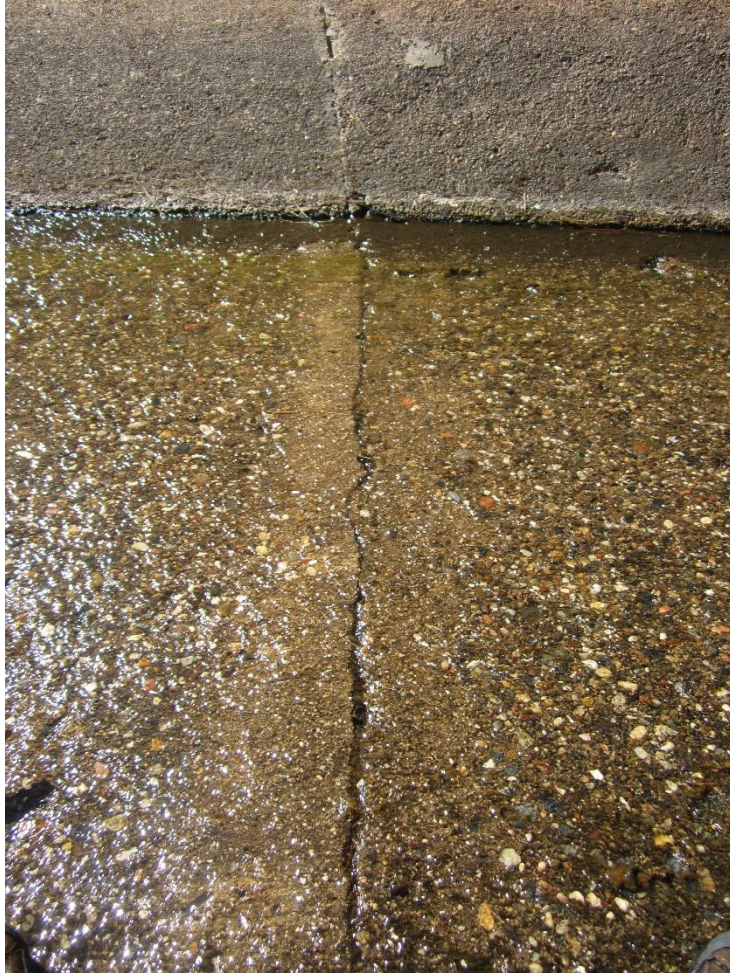
Figure 3-18: Transverse joint at Station 3+25.
