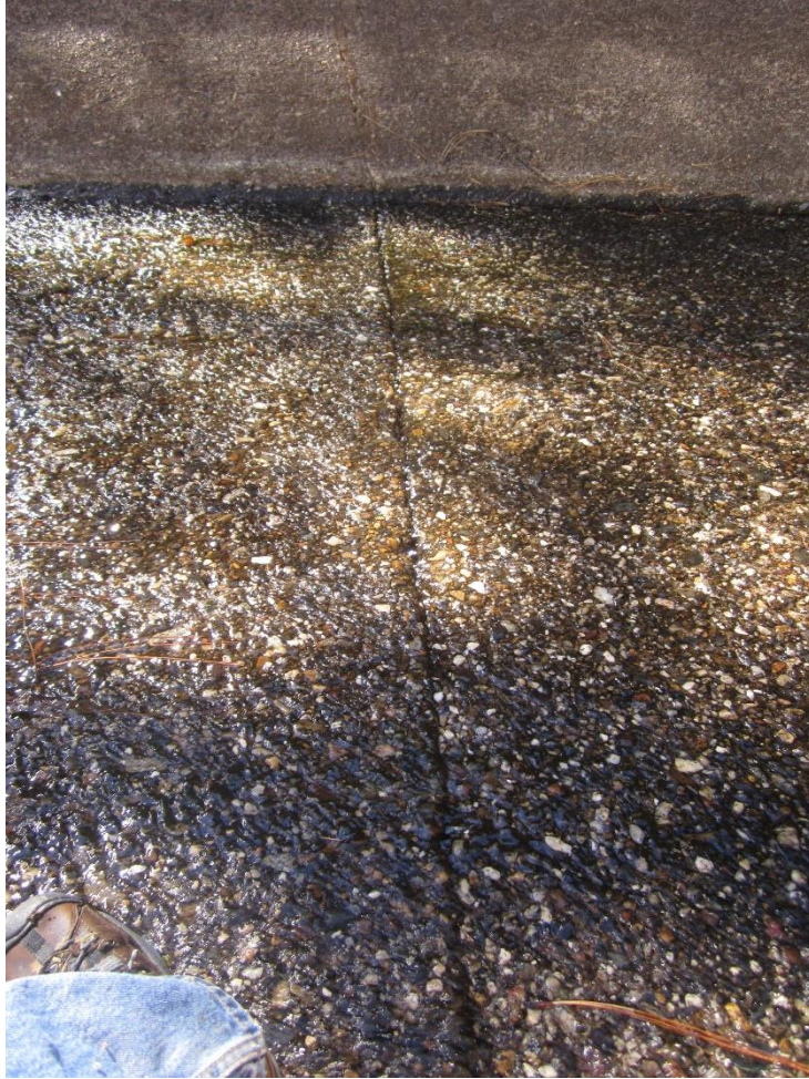
Figure 3-53: Transverse joint at Station 5+00.
