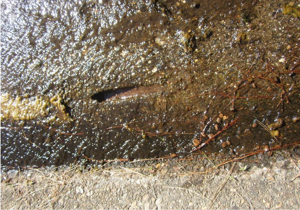
Figure 3-12: Gravel downstream of right blanket drain outlet beyond Station 2+75.
