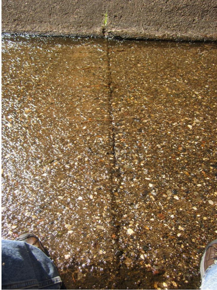
Figure 3-21: Transverse joint at Station 3+50.
