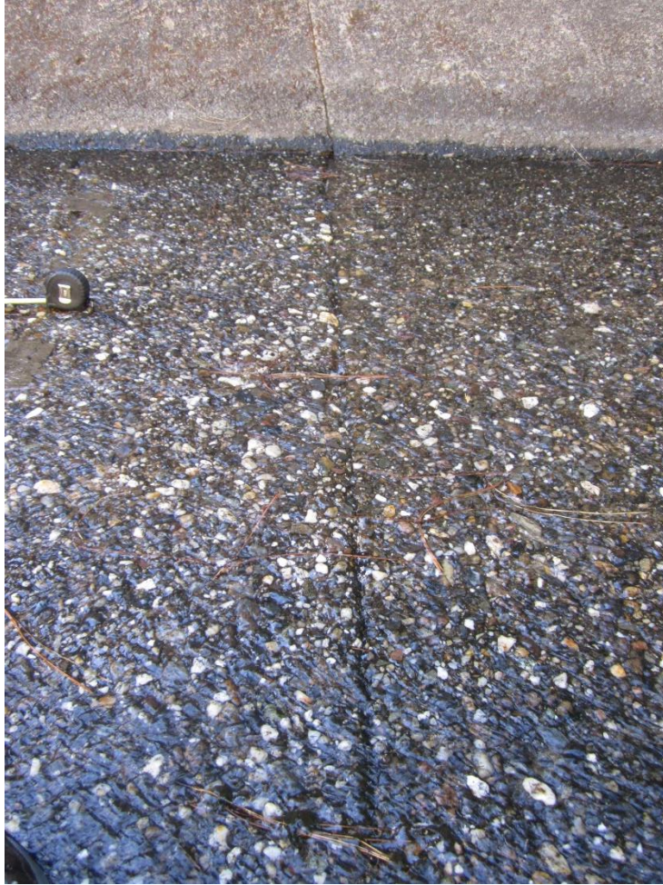
Figure 3-67: Transverse joint at Station 5+50.
