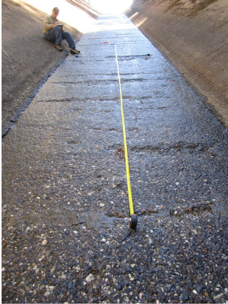
Figure 3-61: Bottom slab between Stations 5+25 and 5+50.
