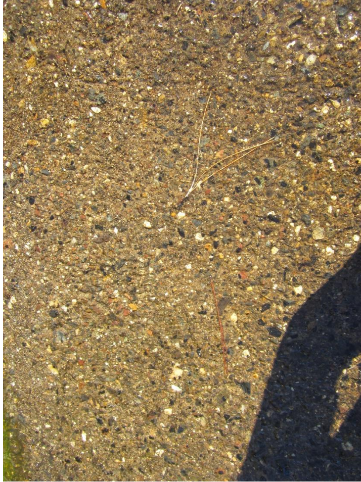
Figure 3-4: Exposed aggregate in bottom slab.
