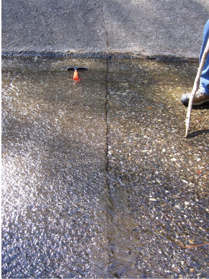
Figure 3-28: Transverse joint at Station 4+00.
