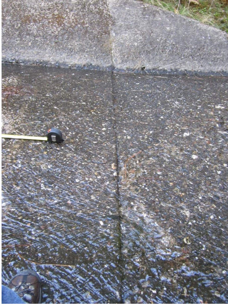
Figure 3-80: Transverse joint at Station 6+00.
