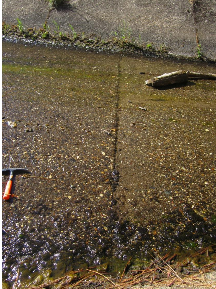
Figure 3-5: Transverse joint at Station 2+25.
