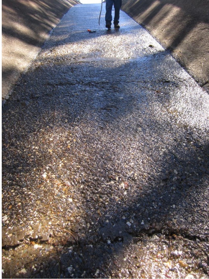
Figure 3-40: Bottom slab between Stations 4+50 and 4+75.
