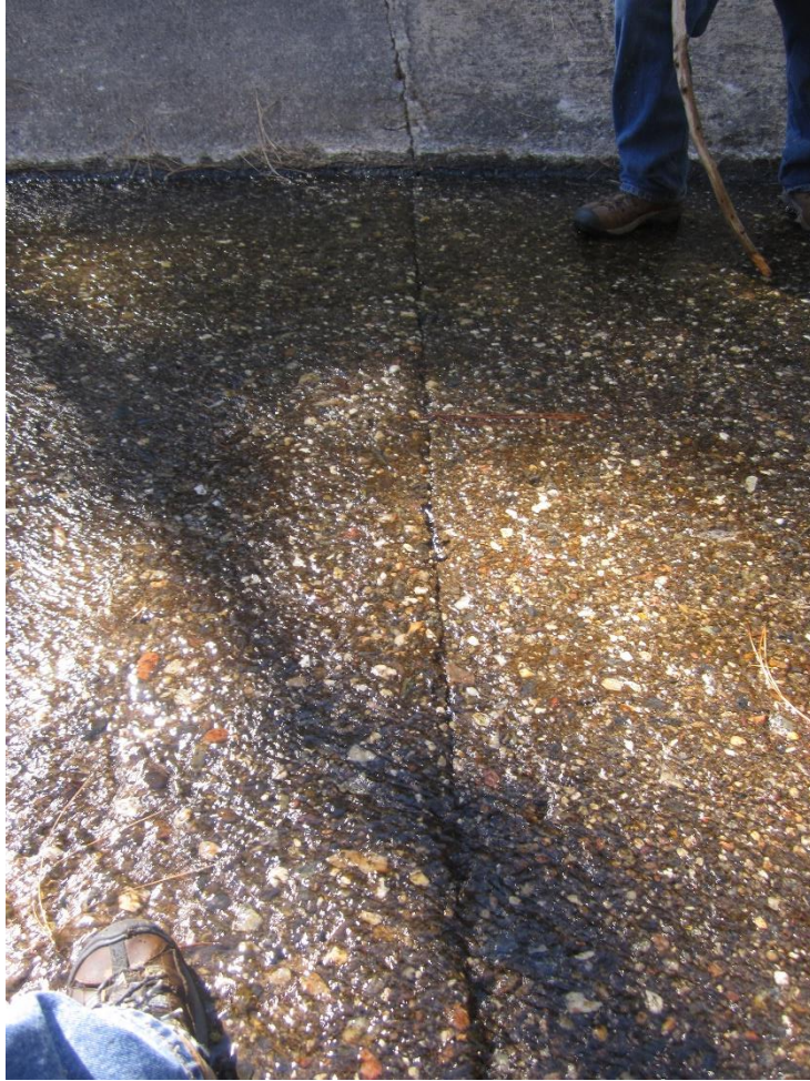
Figure 3-33: Transverse joint at Station 4+25.
