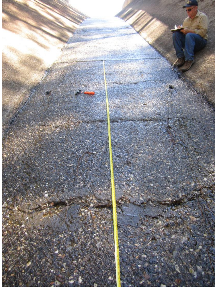
Figure 3-47: Bottom slab between Stations 4+75 and 5+00.
