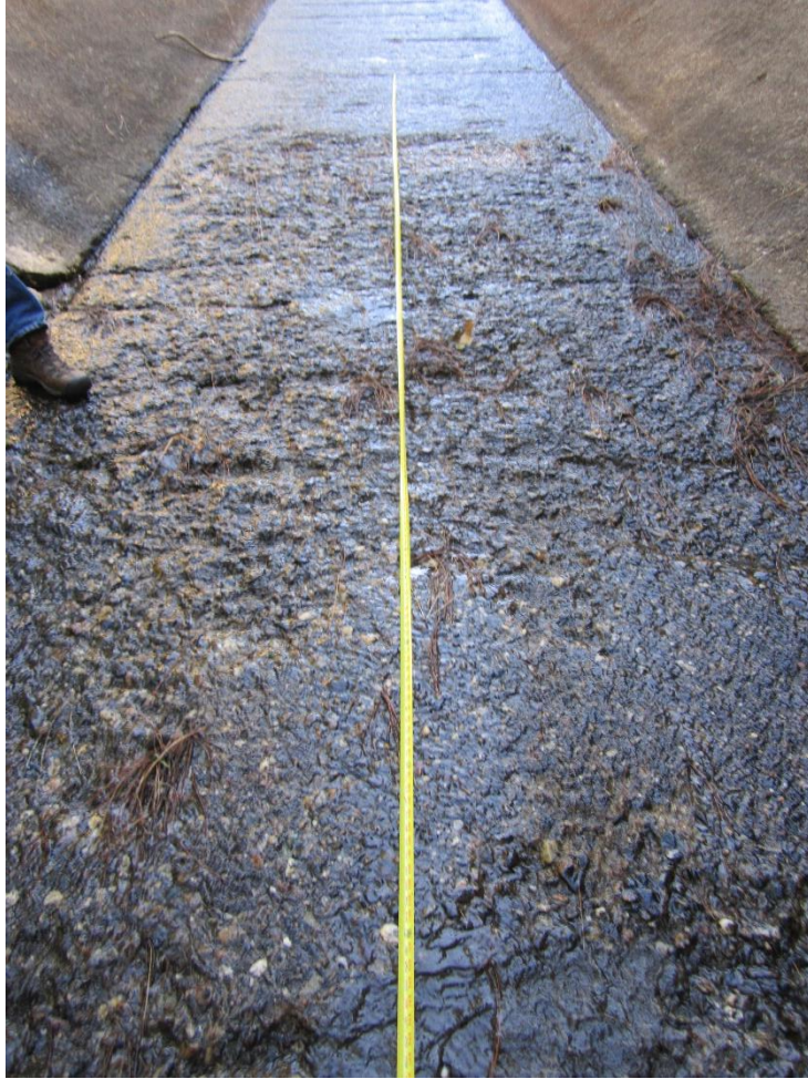
Figure 3-68: Bottom slab between Stations 5+50 and 5+75.
