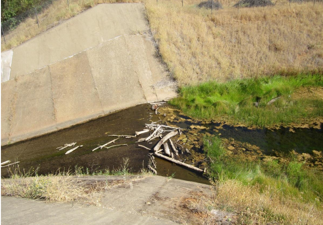
Figure 3-2: Spillway crest with moderate amount of woody debris.
