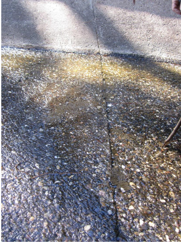
Figure 3-39: Transverse joint at Station 4+50.
