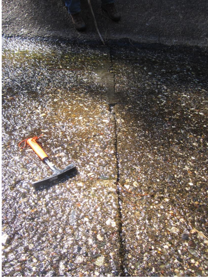
Figure 3-46: Transverse joint at Station 4+75.
