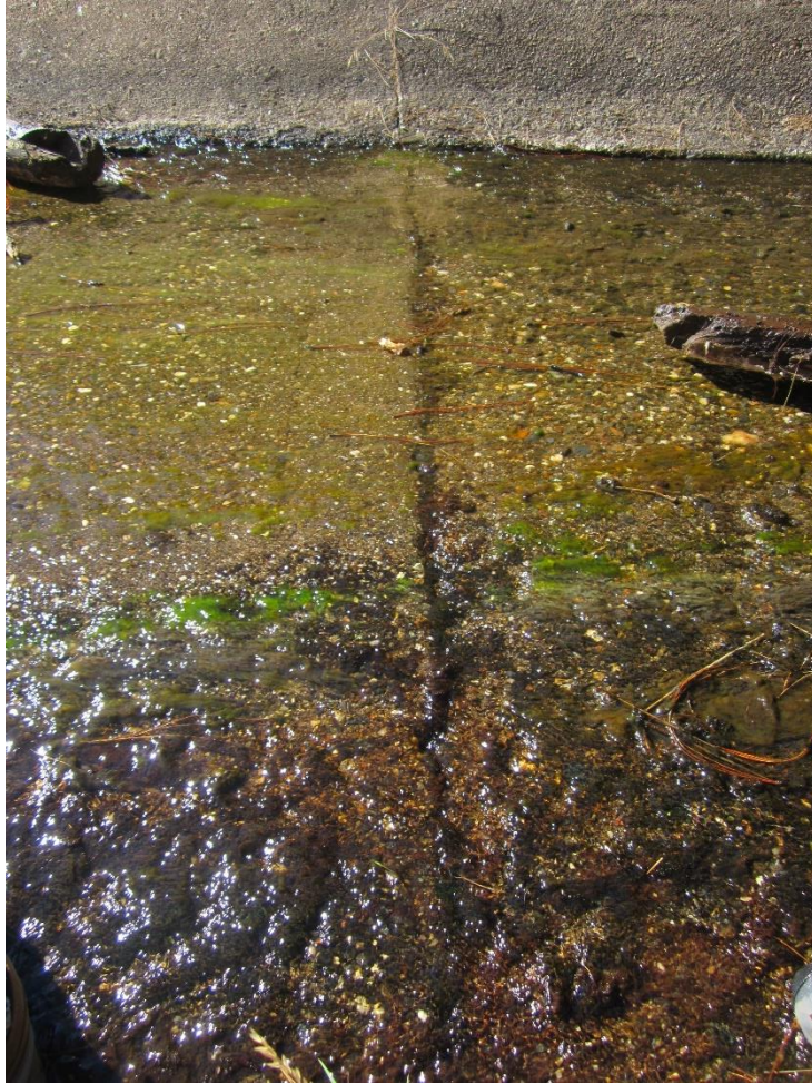
Figure 3-7: Transverse joint at Station 2+50.
