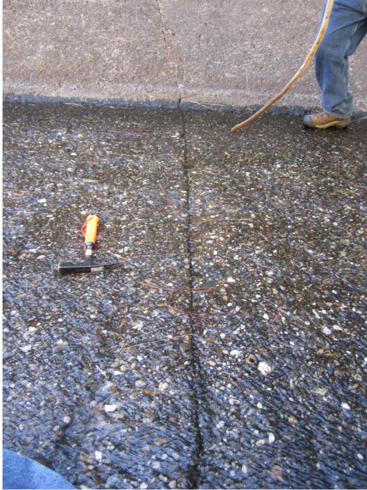
Figure 3-60: Transverse joint at Station 5+25.
