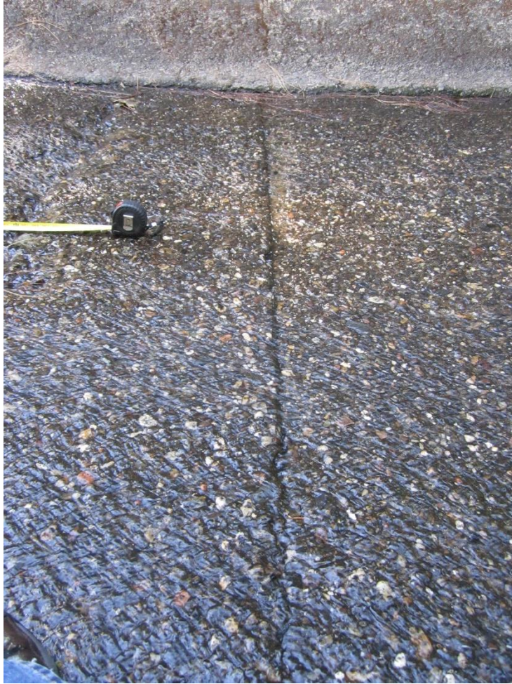
Figure 3-73: Transverse joint at Station 5+75.
