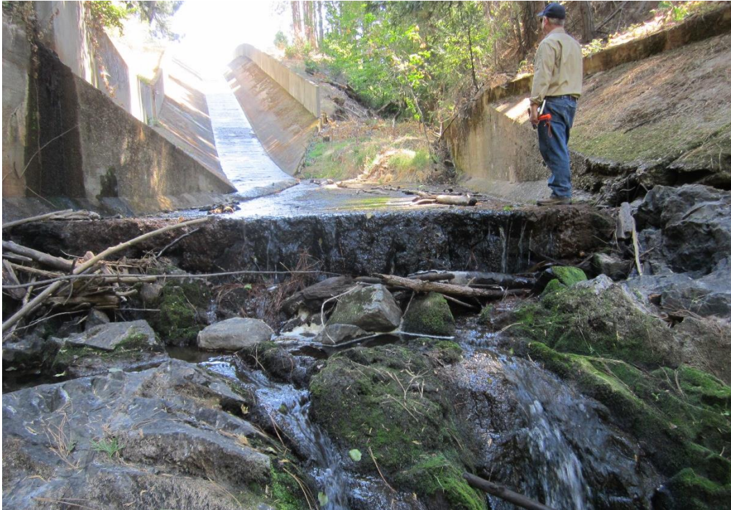
Figure 3-82: End of chute bottom slab at approximately Station 6+70.
